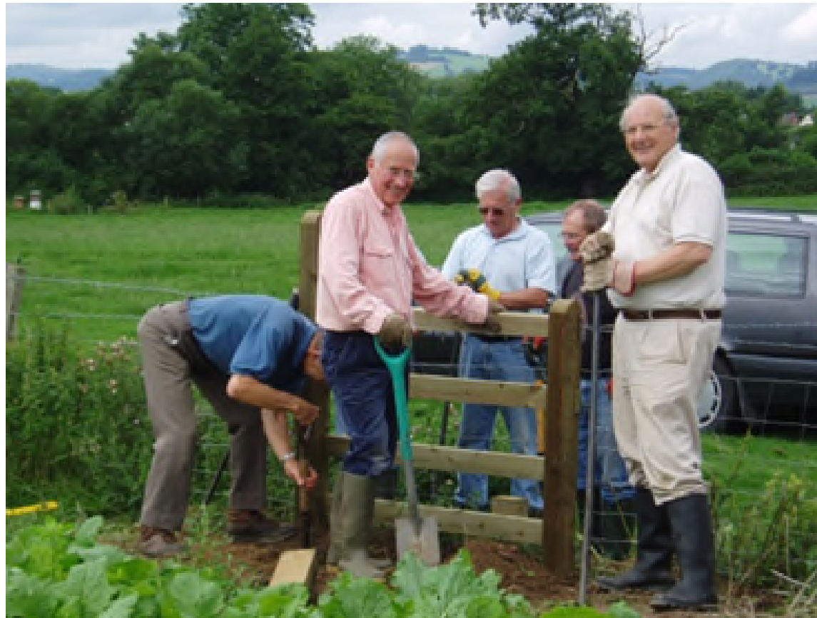
Installing a stile
